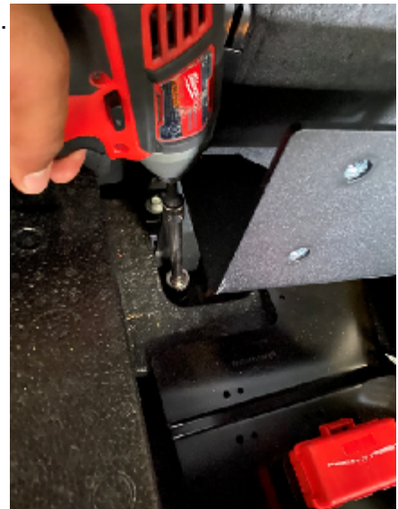
Fig.8 IMAGE FROM REAR END INSTALLED PASSENGER SIDE LOWER BRACKET
