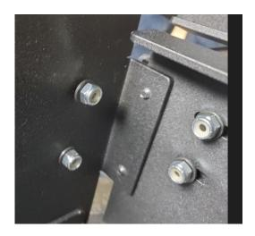
d) Add 10-24 screws, washers and lock nuts to attach the side brackets to the vaults and leave them loose.
